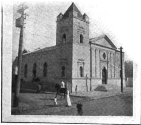
Our Model Baptist Church in Ponce. Such houses command respect and give us proper standing and equipment
