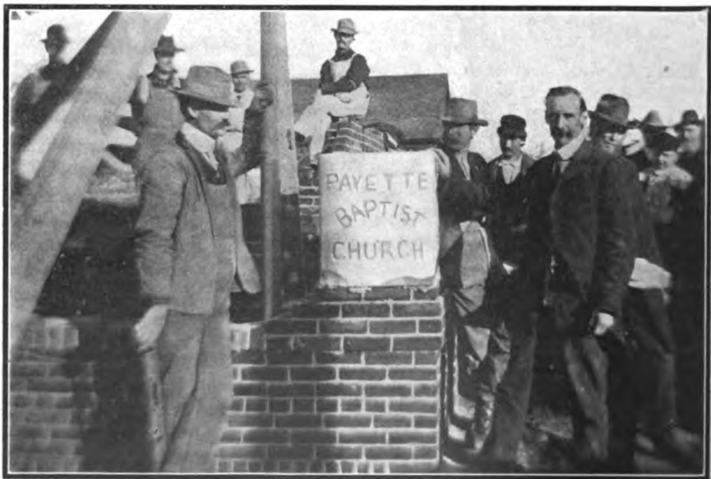
PASTOR AND MEMBERS LAYING THE CORNER STONE
