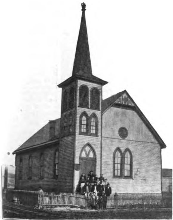
FIRST SLOVAK CHURCH IN NORTH AMERICA, AT CREIGHTON, PA.
