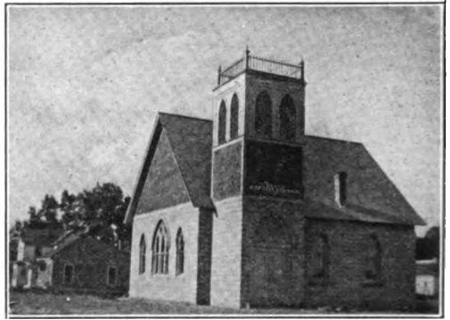
FIRST CHURCH IN FALLON, NEV.; CONCRETE BLOCKS, SEATS 200. COST $3,240; BEST BUILDING IN NEW TOWN; AIDED BY CHURCH EDIFICE DEPARTMENT
