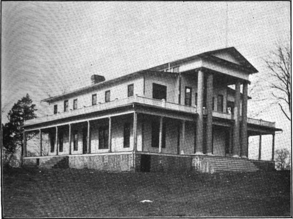
THE NEW BUILDING OF ROGER WILLIAMS UNIVERSITY AT NASHVILLE
