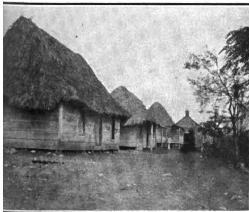
FIRST BUILDING IS A PUBLIC SCHOOL
