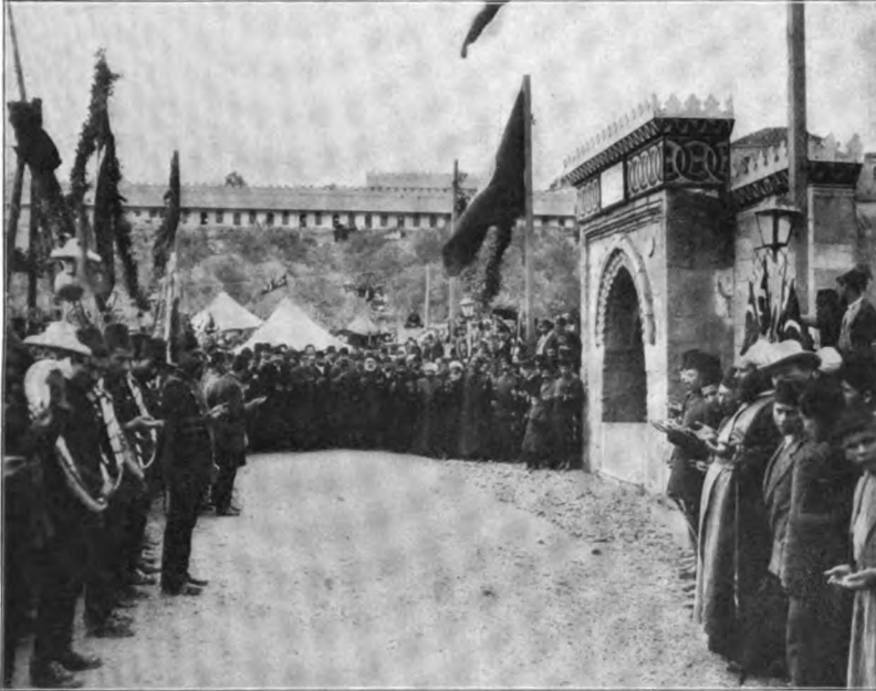
THE INAUGURATION OF THE NEW WATER SUPPLY AT THE FOUNTAIN ON THE JERUSALEM-BETHLEHEM ROAD.
